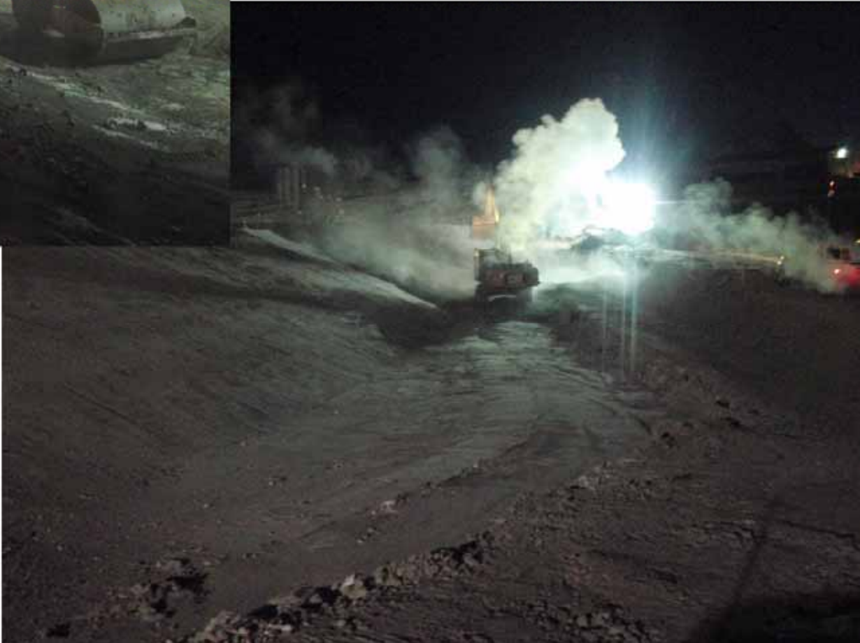
Photo 15: ~NE view down over inflection point of the dam towards the Overliner placement at the N The area show in this picture was cleaned of snow and large debris. The area south of (or behind) this picture still requires notable snow clearing.
