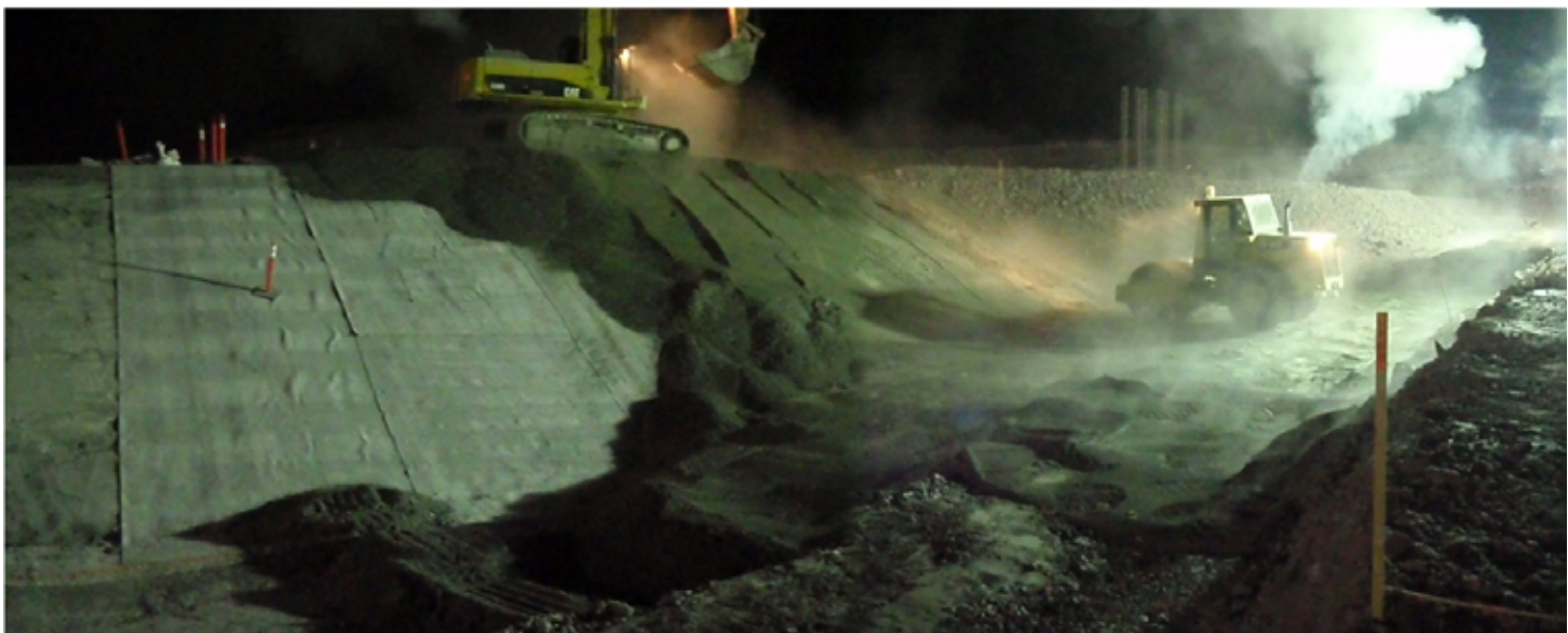
Photo 13: ~NNW stitched panoramic view of excavator spreading Overliner material. As noted by dayshift one panel row of GCL had a seam that was overlapped on the upstream slope. These GCL panels can be observed in the left of this picture.
