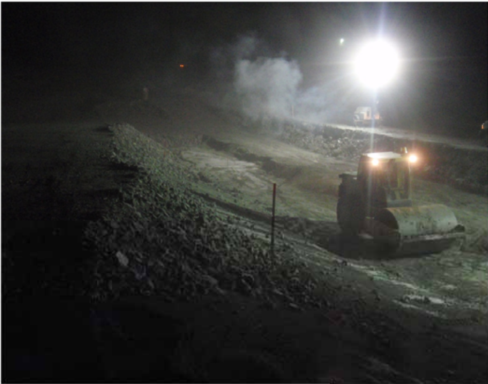
Photo 14: ~ NE view from 1+40 of Transition material placed on dayshift. Note that the majority of the placed transition material was placed first on the crest of the dam. Additional material required on the upstream dam slope from ~ 1+95 to 1+60.
