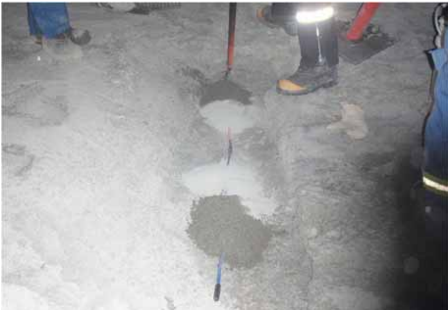
Photo 9: The final three exposed beads on thermistor cables ND-HTS-060-33.5 being installed in FCM.
