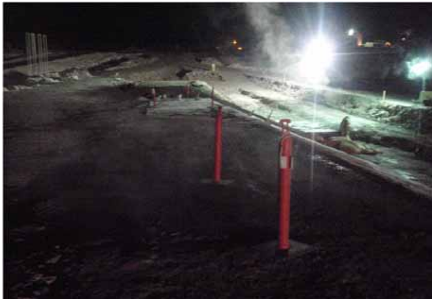
Photo 8: Area on the top crest of the dam, around 1+05 to 1+20, that was built up on the downstream and upstream crest with a small lift of material (~0.1 to 0.15m left).
