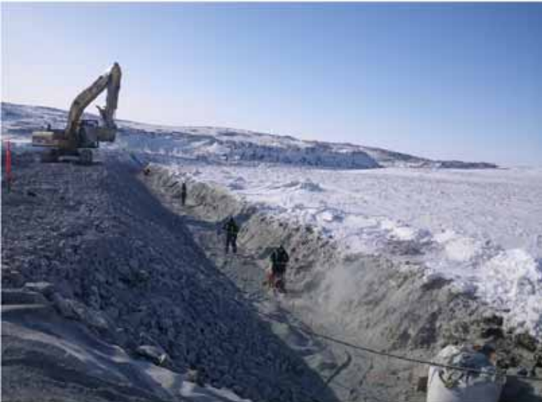
Photo 7: plate tamping the crush on the floor of the Diversion Berm, just west of 1+60. Photo looking west.
