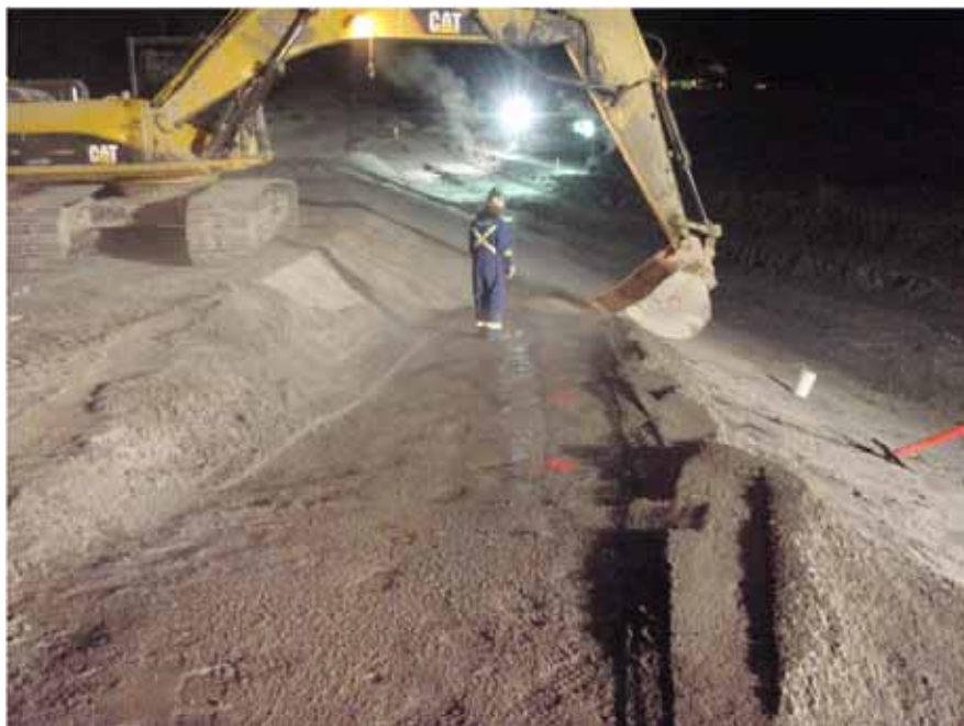
Photo 10: View of lift of FCM placed in underbuilt SSE corner of the core. Note the paint marks outlining the crest that this lift was required to be cut back to after being overbuilt and packed.
