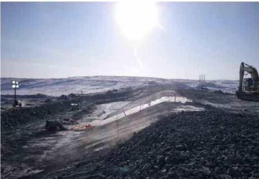
Photo 2: looking south west along the dam stranding on the placed transition material.
