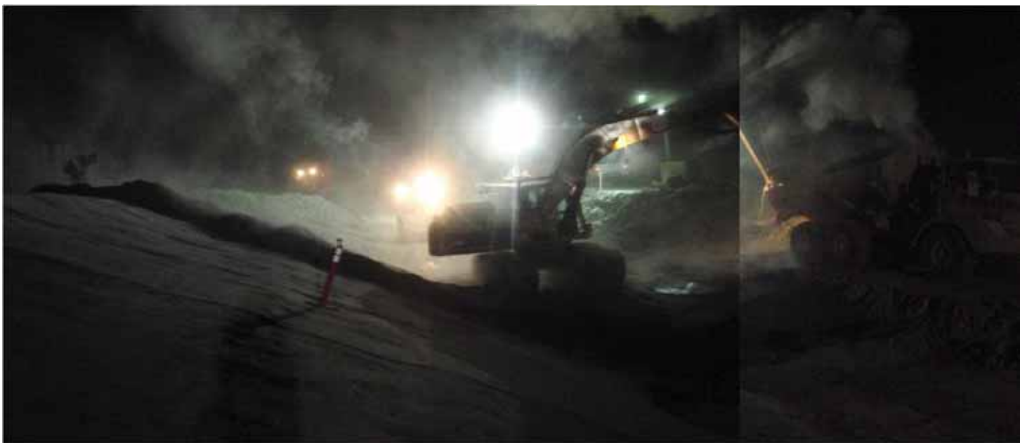
Photo 12: ~ NNE stitched panoramic view of 330 excavator placing and 730 truck dumping Overliner material around 1+30.
