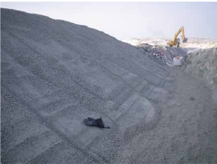
Photo 4: Underliner crush material placed in Diversion Berm. Photo looking west, mega bag is ~1+60
