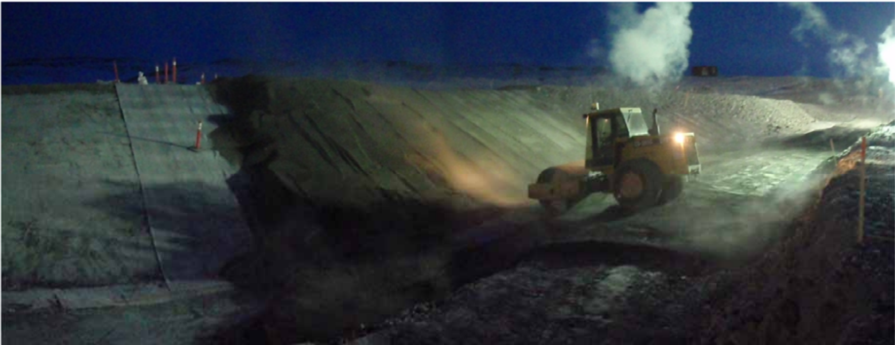
Photo 16: Packer starting to compacted the side slopes around 1+30 to 1+20 (stitched panoramic
