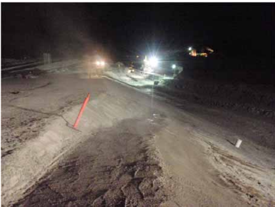
Photo 11: ~NE view of SSE underbuilt corner of the core. Photo taken after final sloping completed. Note that on the order of 3 lifts remain to be placed in this underbuilt sliver.
