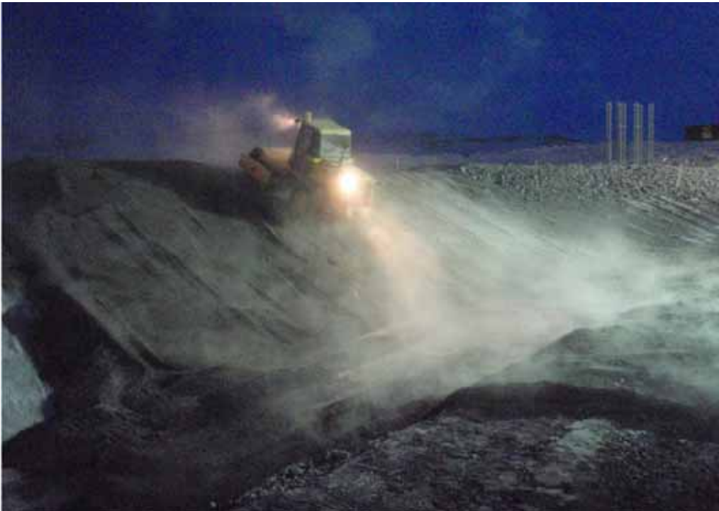
Photo 17: 10 ton vibrator packer vibratory rolling the upstream slope.
